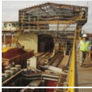
Dampier Port Upgrade
