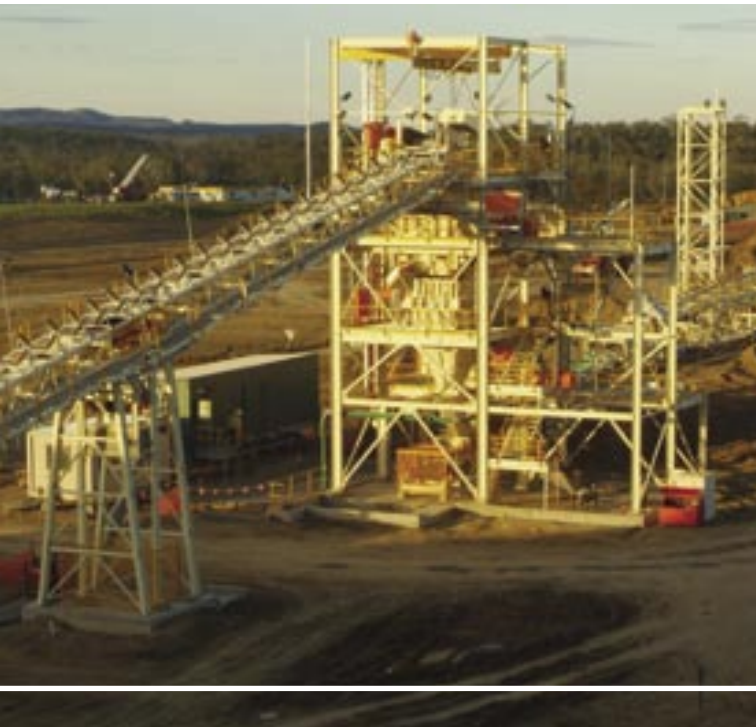
Sizing Station, Rolleston Coal Handling Facility
